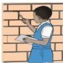
*Fig. 2.8. Pupil using a jointer*
